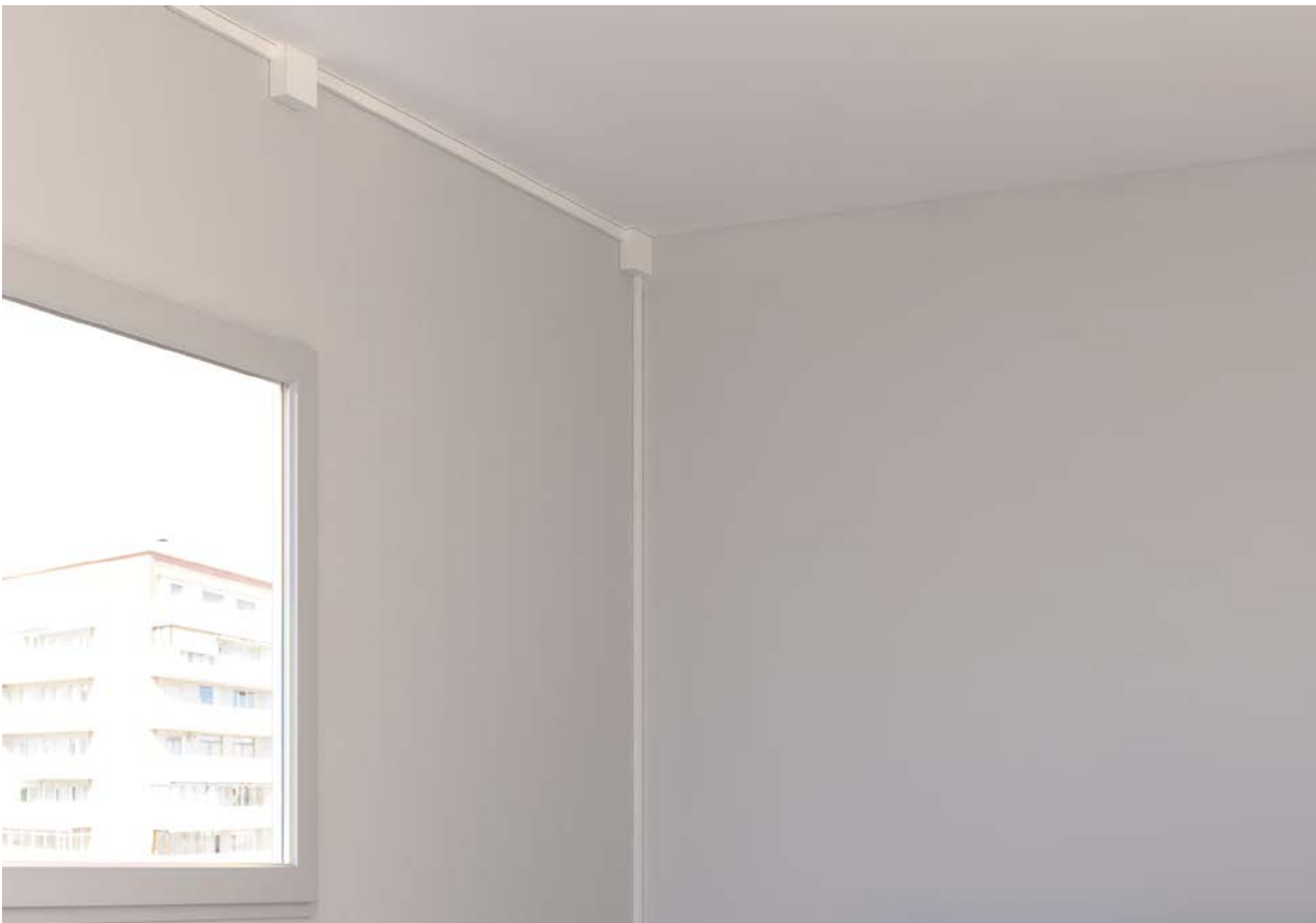
Apartment building renovation
